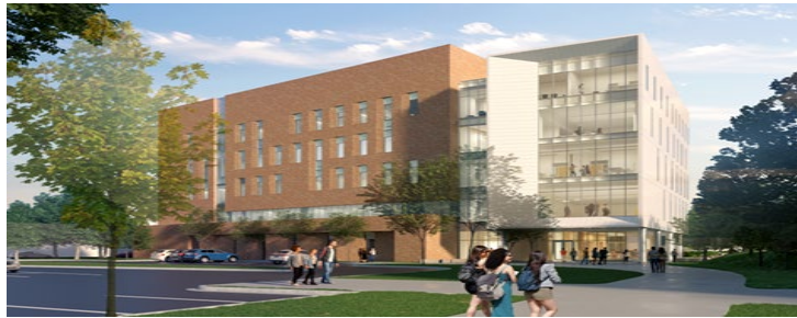
School of Nursing $100MM (~91,000 sf) Under Construction
