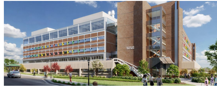
Gant Building Renovations $279MM for Phases 1 - 3 (310,000 sf) Phase 1 & 2 Complete Phase 3 is Under Construction
