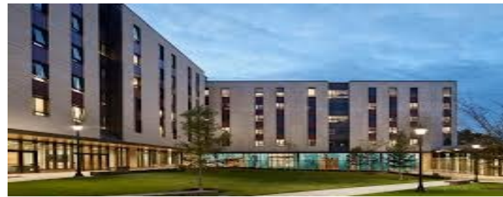
Connecticut Residence Hall & Dining Facility $215MM (~280,000 sf) Opened- Fall 2024
